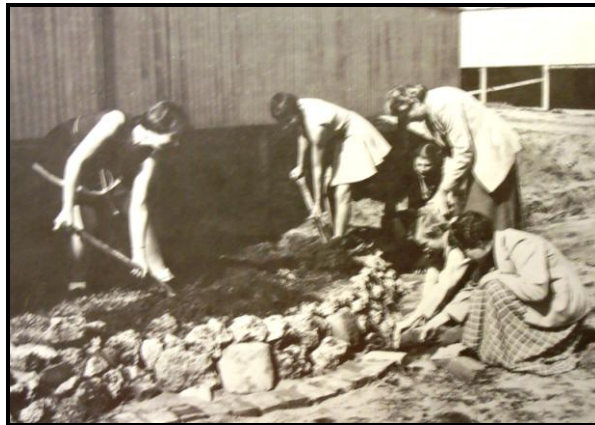
Fig. 28 "The grounds were the real problem ..." c. 1955 228
